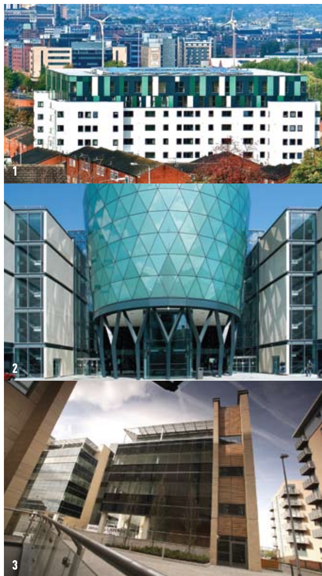
1 Greenhouse is one of the UK's most environmentally sound developments 2 Rose Bowl achieved BREEAM excellent rating 3 The Highways Agency took a prelet on Lateral office building
